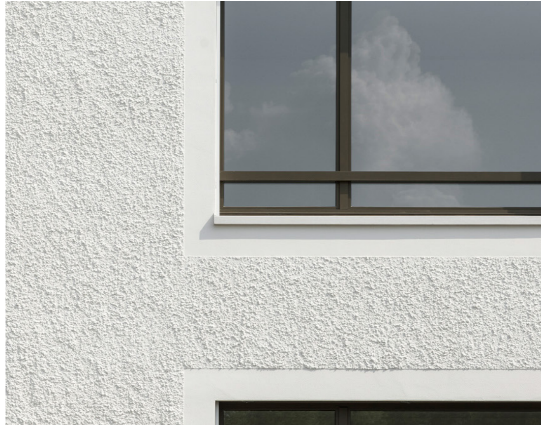
Fig. 50 Rough / Smooth Render Detailing
