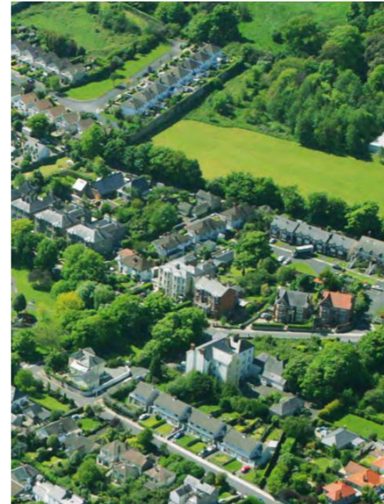
Fig. 15 Traditional House with Two Storey Bay Window
