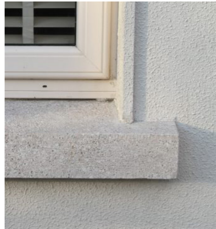
Fig. 49 Extended Stone Sills, Capping, Base
