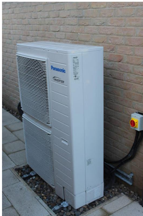
Fig. 5.4 – Typical Air Source Heat Pump Installation
