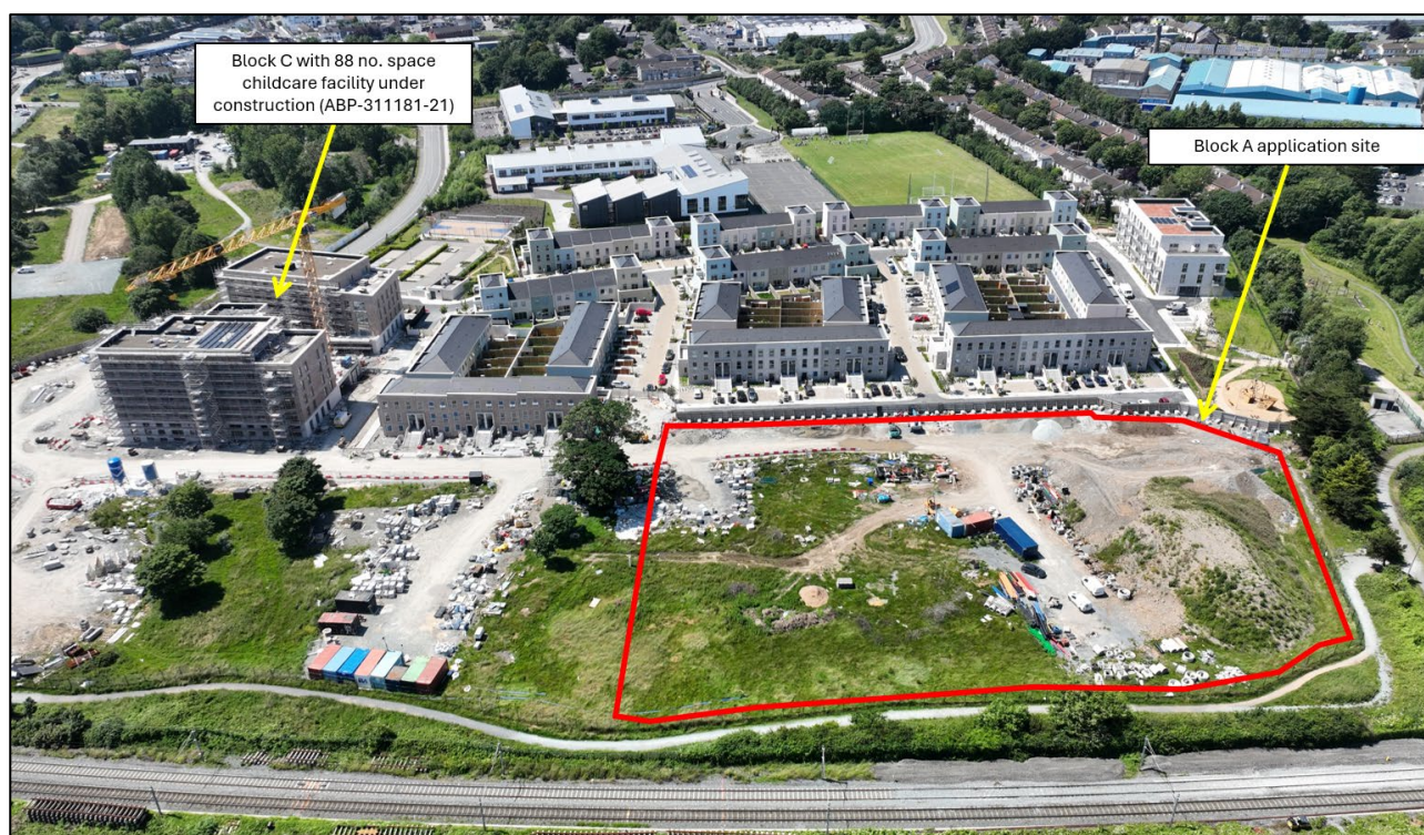
Figure 2-2: Sea Gardens Phase 1 lands with childcare facility under construction
